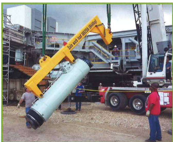
06 JEL- cylinder handled with the lifting fixture
